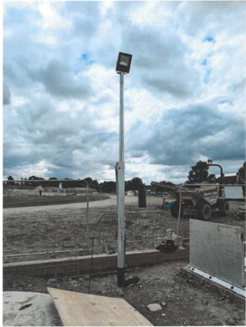
Civils have installed Lamp Column – PDAS to fit floodlight and wire up to Kiosk
