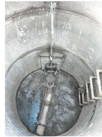
Civils have installed Inlet Manhole Penstock Valve, Spindle and Top Box
