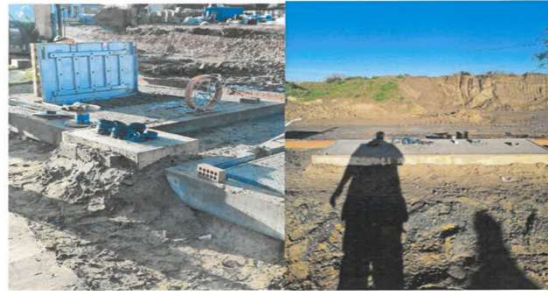
Civils have installed Inlet Manhole Penstock Valve, Spindle and Top Box
